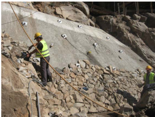
Photograph 1 – Coating the concrete structures
