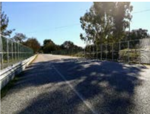
Barriers to elevate the flight of flying species, in particular bats, nocturnal birds of prey and passerine birds
