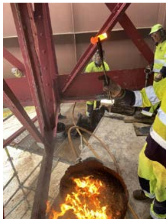
Bridge Brigade works
