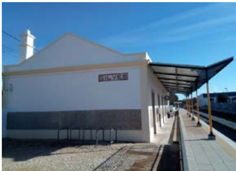
Improvement of Silves station
