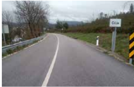
After the works
