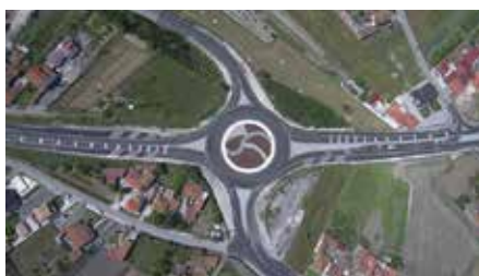
After the works
