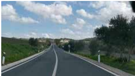
After the works
