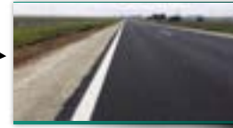
ER2, km 603+000 and km 609+000. Improvement. IPV2018
